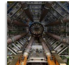
Box build and cabling of CERN power systems
